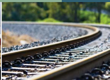
WestNet Rail, Australia
